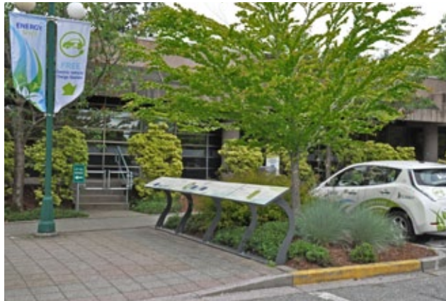
Top. Edible Canada EVSE Installation, BC, Canada
