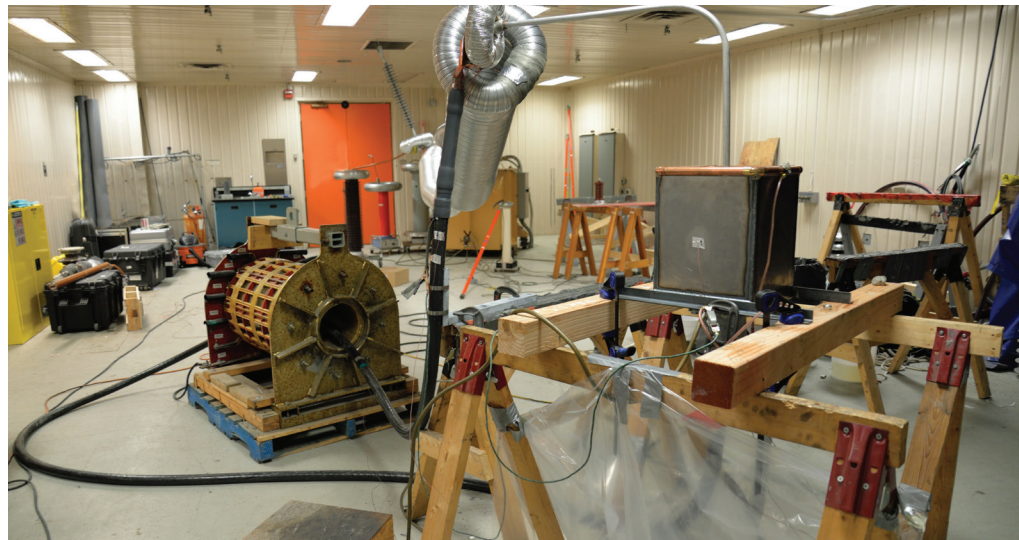
High voltage cable testing in the MV (medium voltage) Lab
