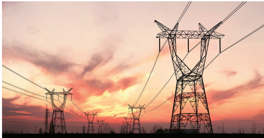
Asset management of transmission line overhead components
