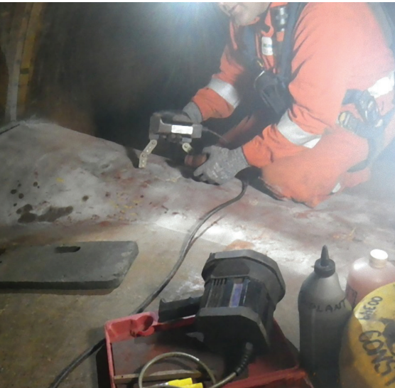
NDT inspection of turbine inlet valve
