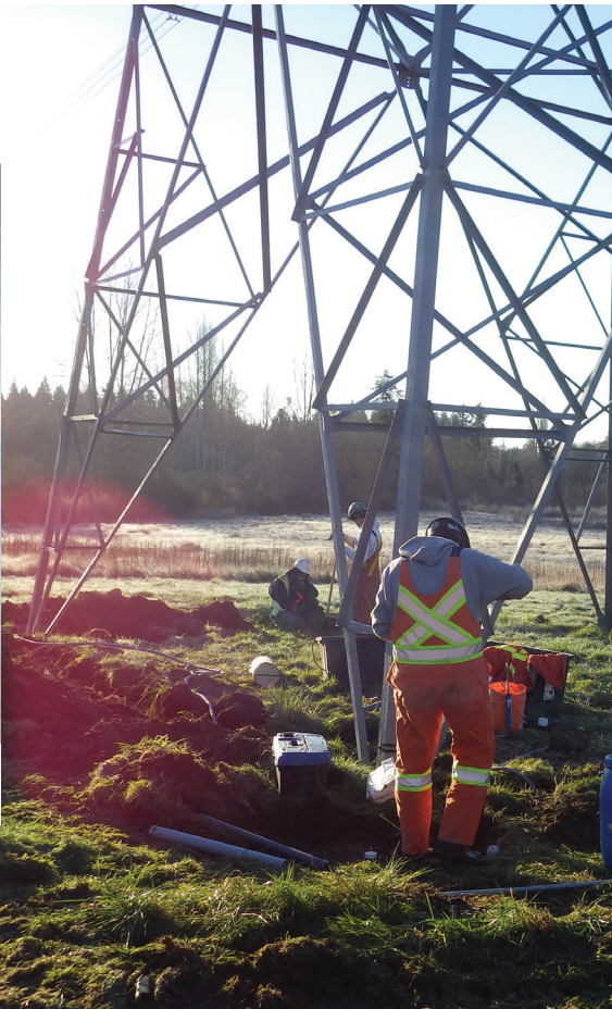
Installation of SACP system
