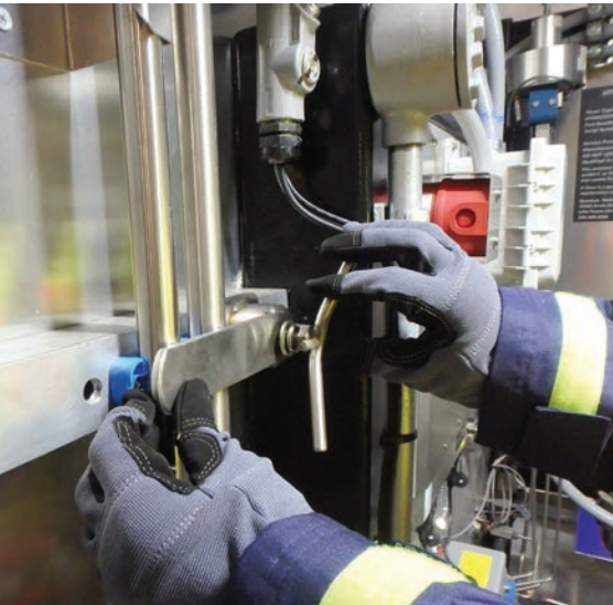
Hydrogen station fabrication
